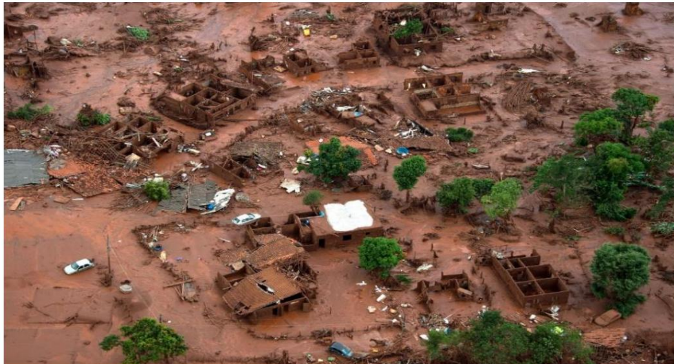
Figure 03: Aerial image of the Bento Rodrigues district, after the Fundão dam collapse.
