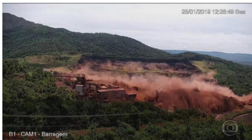
Figure 04: Rupture of the Vale dam at the Córrego do Feijão Mine, in Brumadinho.
