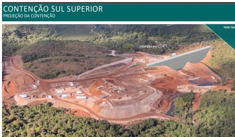
Figure 07 – Construction of the concrete containment located 6 km downstream of the Sul Superior dam, in Baron of Cocais.
