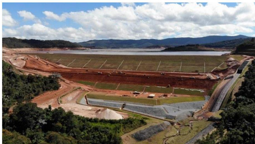
Figure 01 – Raising of the Itabiruçu Dam Itabira / MG.
