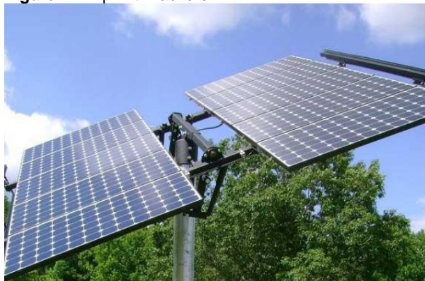
Figure 4 – Tip Tilt Trackers
