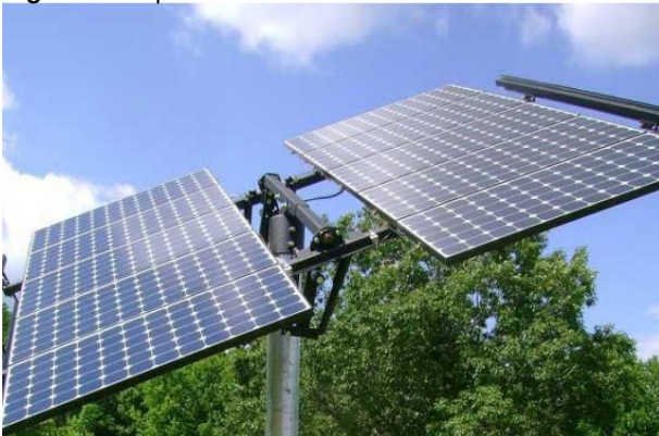
Figure 4 – Tip Tilt Trackers
