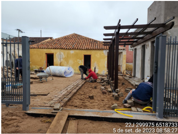
Situation of the patio area recorded in September 2023, with changes to the soil: removal and replacement of cobblestone and placement of sand backfill layer
