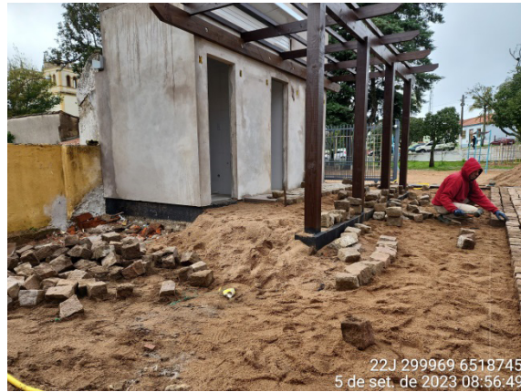
Status of the patio area recorded in September 2023. Pergola and beam added to the structure bathroom area, layer of sand embankment 20cm and laying cobblestones
