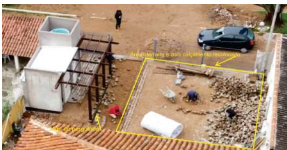
Situation of the patio area recorded in September 2023, with changes to the soil: removal and replacement of cobblestone and placement of sand backfill layer
