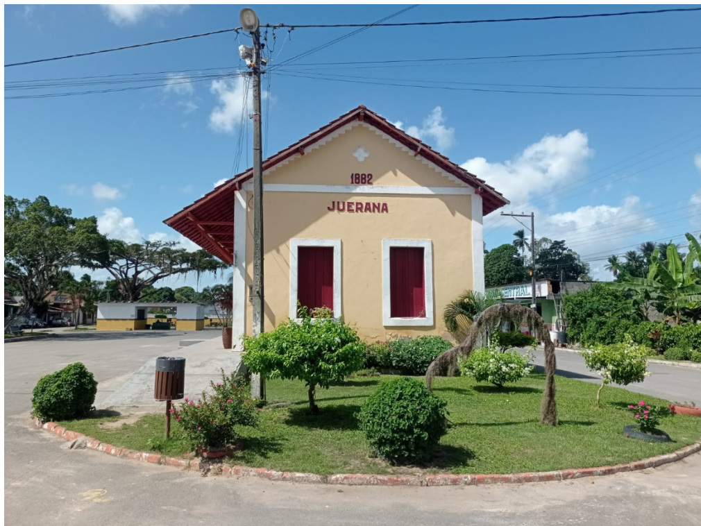
Figure 3 - Bahia and Minas Railway Station in Juerana
